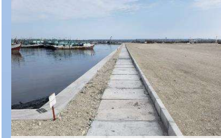
Pek Retaining Wall
